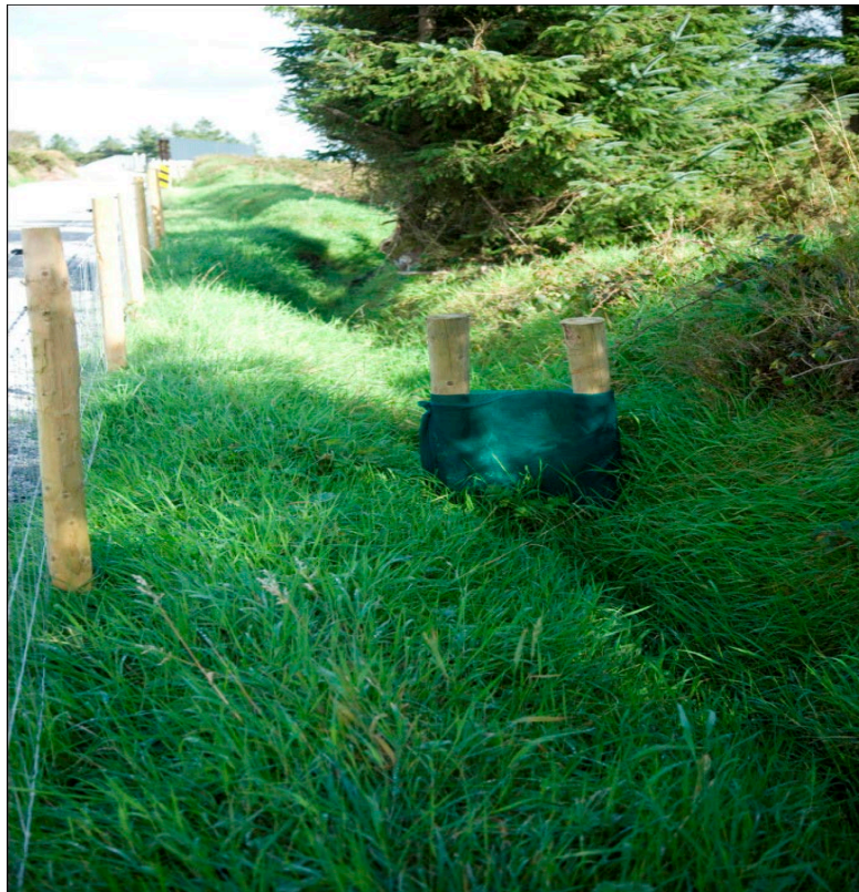
Figure 4-5: Silt Trap across Grassed Swale
