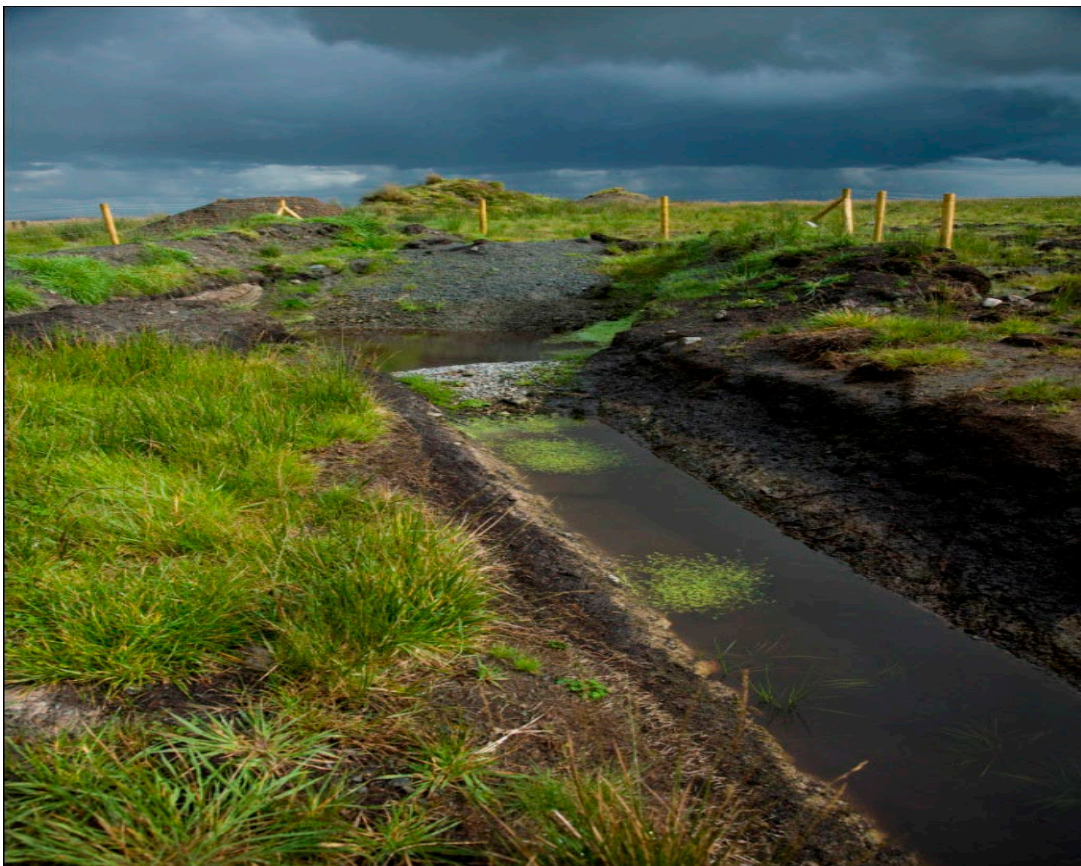
Figure 4-3: Swale draining to Stilling pond
