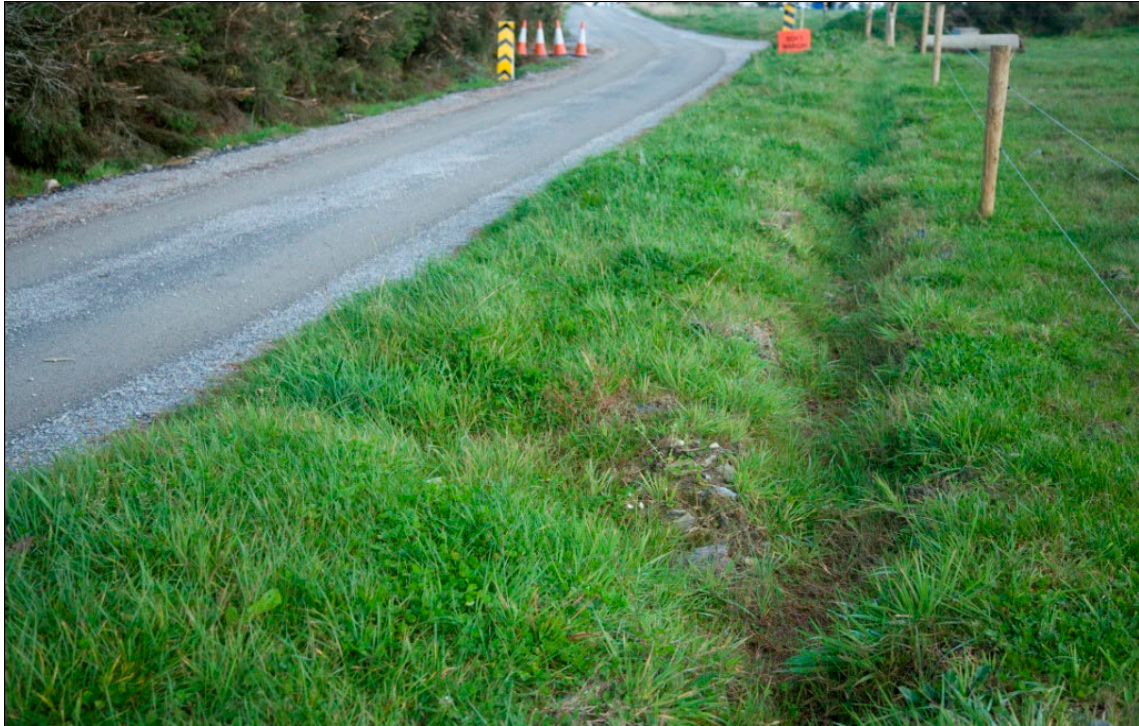
Figure 4-2: Grassed Swale along access track
