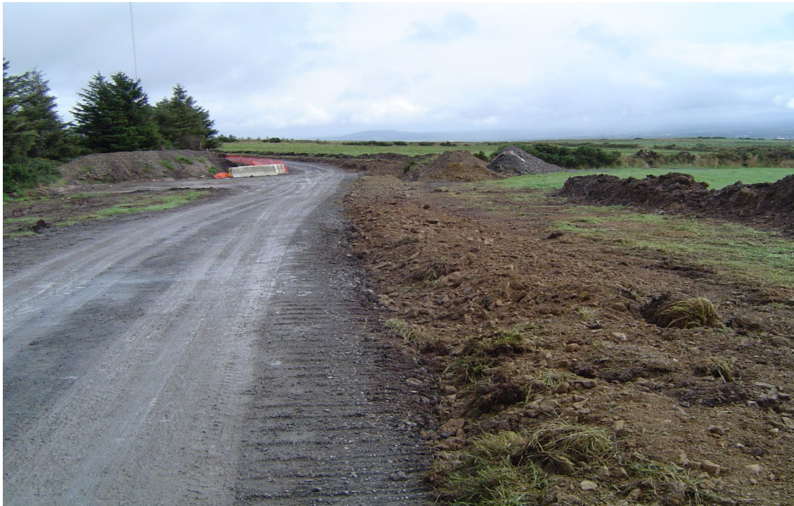
Figure 4-8: Backfill over Cable Trench
