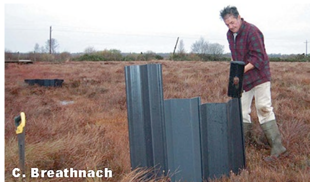
Plate 4-1: Plastic piling being installed within IPCC bog
