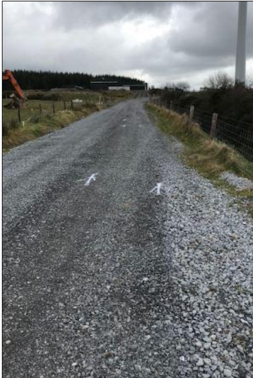
Figure 3.7: Typical Access Track
