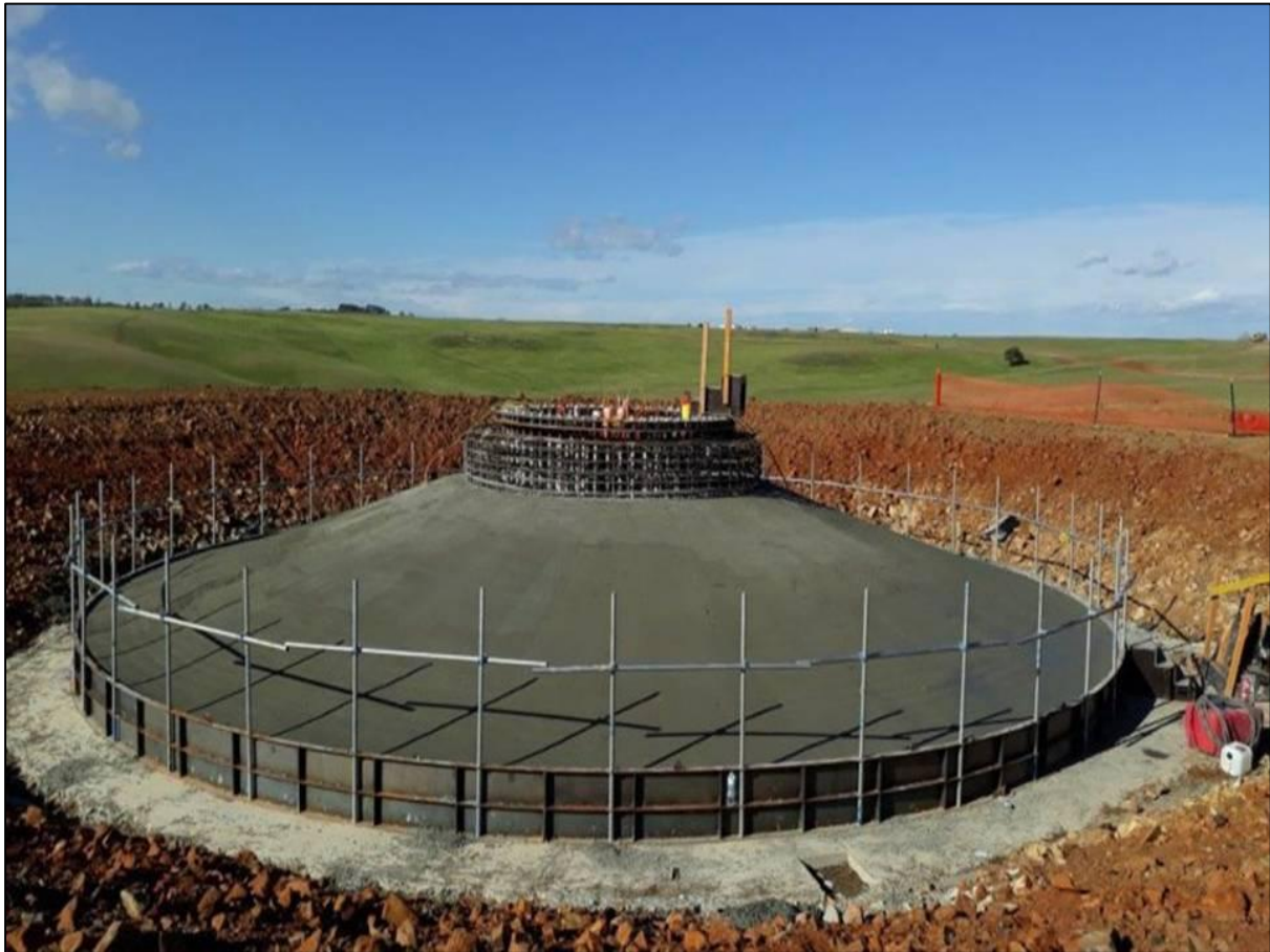
Figure 3.6: Typical Turbine Foundation
