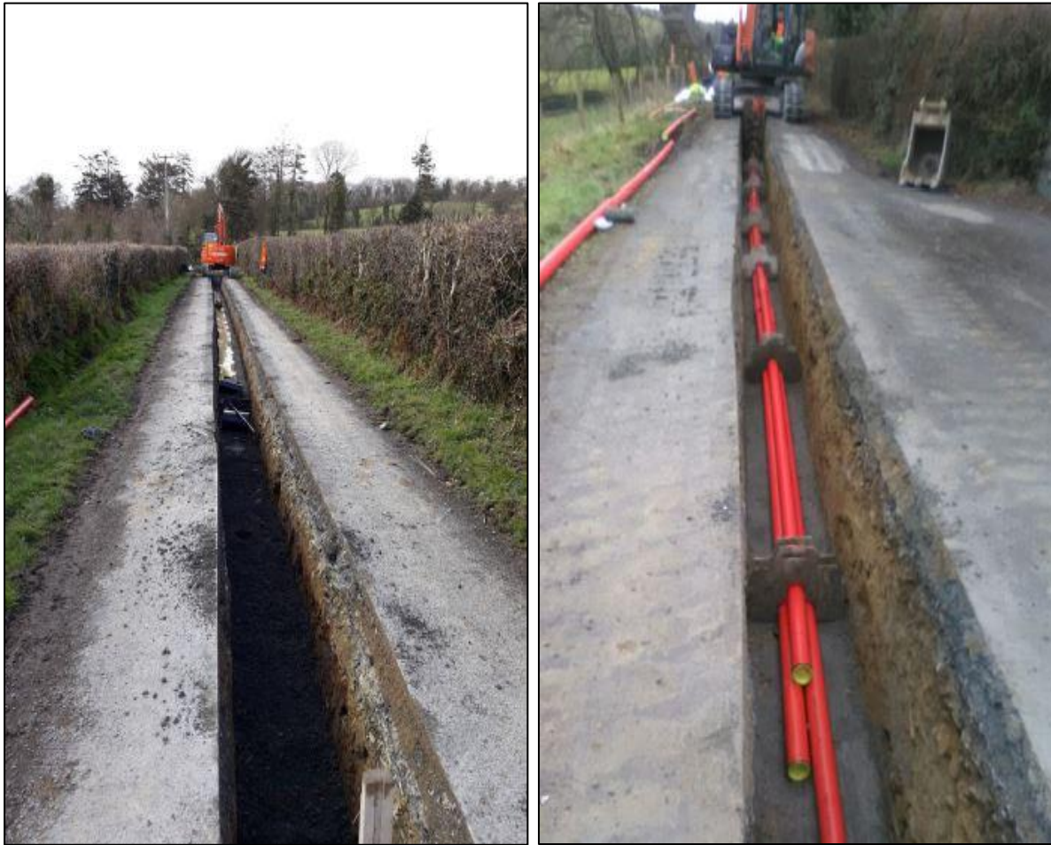
Figures 3.8 and 3.9: Typical Trench Construction
