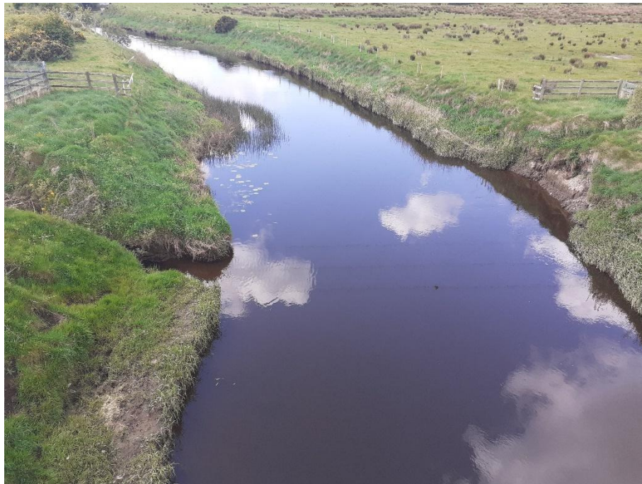
Plate 16 - Site 11 (FH6) - Fish habitat survey facing upstream deep glide
